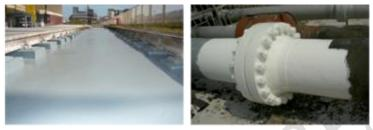
coating. Where the concrete is dry but highly porous, it is recommended to condition with *BC 909 PP*.
