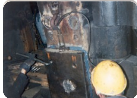
Steel Mill Hammer Foundation
